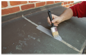
• Protection against corrosion on lead and zinc
