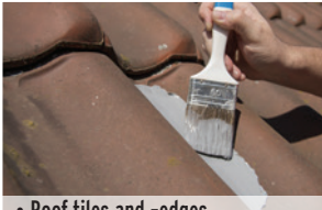
• Roof tiles and -edges
