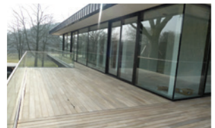
• Coating below terraces
